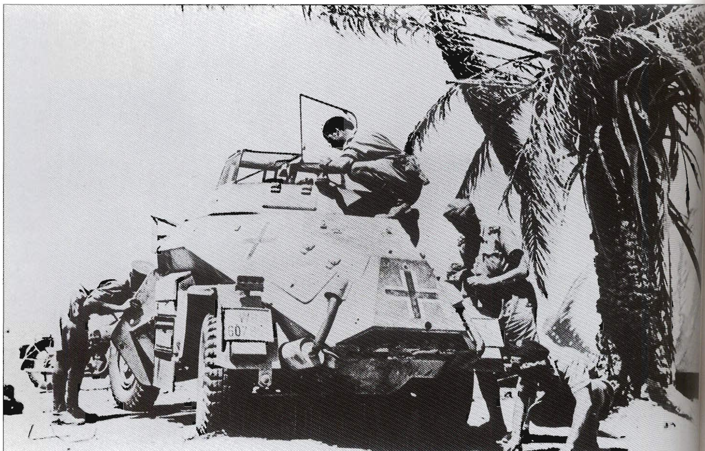
British soldiers inspect another Sd.Kfz. 222 that looks relatively intact however note the penetration hole in the front plate next to the storage box. It is similarly marked to the other vehicle but the remnants of a tactical marking appear on the left side engine compartment access door. The vehicle registration number - WH 607858 - is painted on the front and rear and a faint 15. Panzer-Division emblem can be seen on the left mudguard between the Nottel light base and headlight.
