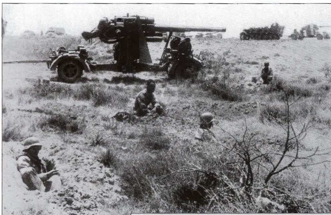
The crew of this 8.8cm Flak rest in their foxholes during a lull in fighting. The gun is still limbered on trailer to allow it to be easily moved to a different location. After firing, the muzzle blast raised a large cloud of dust that permitted the enemy to quickly spot their location and begin suppressing artillery fire.
